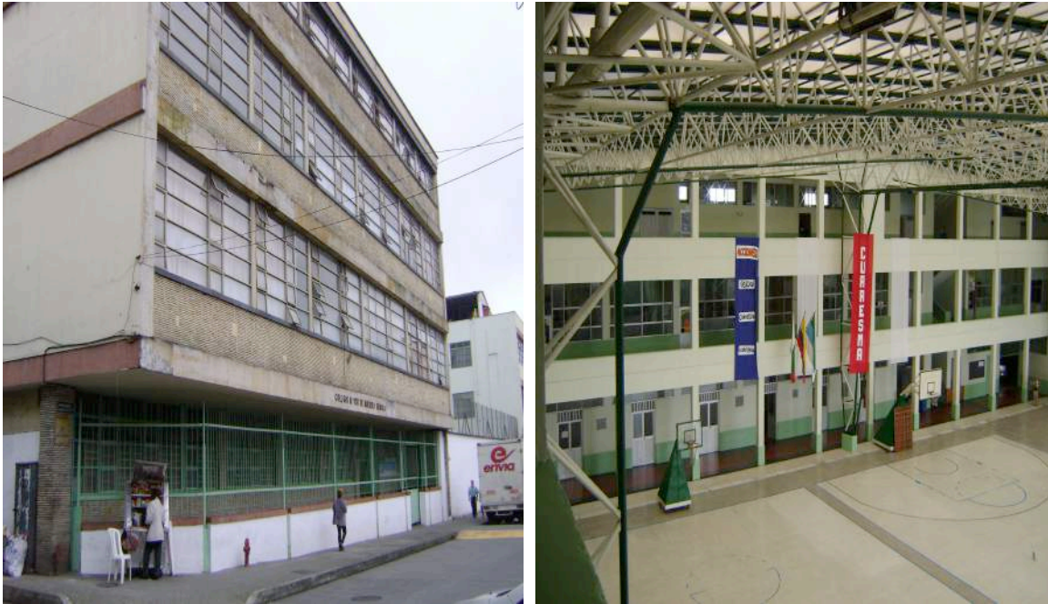
Figures 2 and 3. School's entrance and main patio/sports court. Photos by author.
